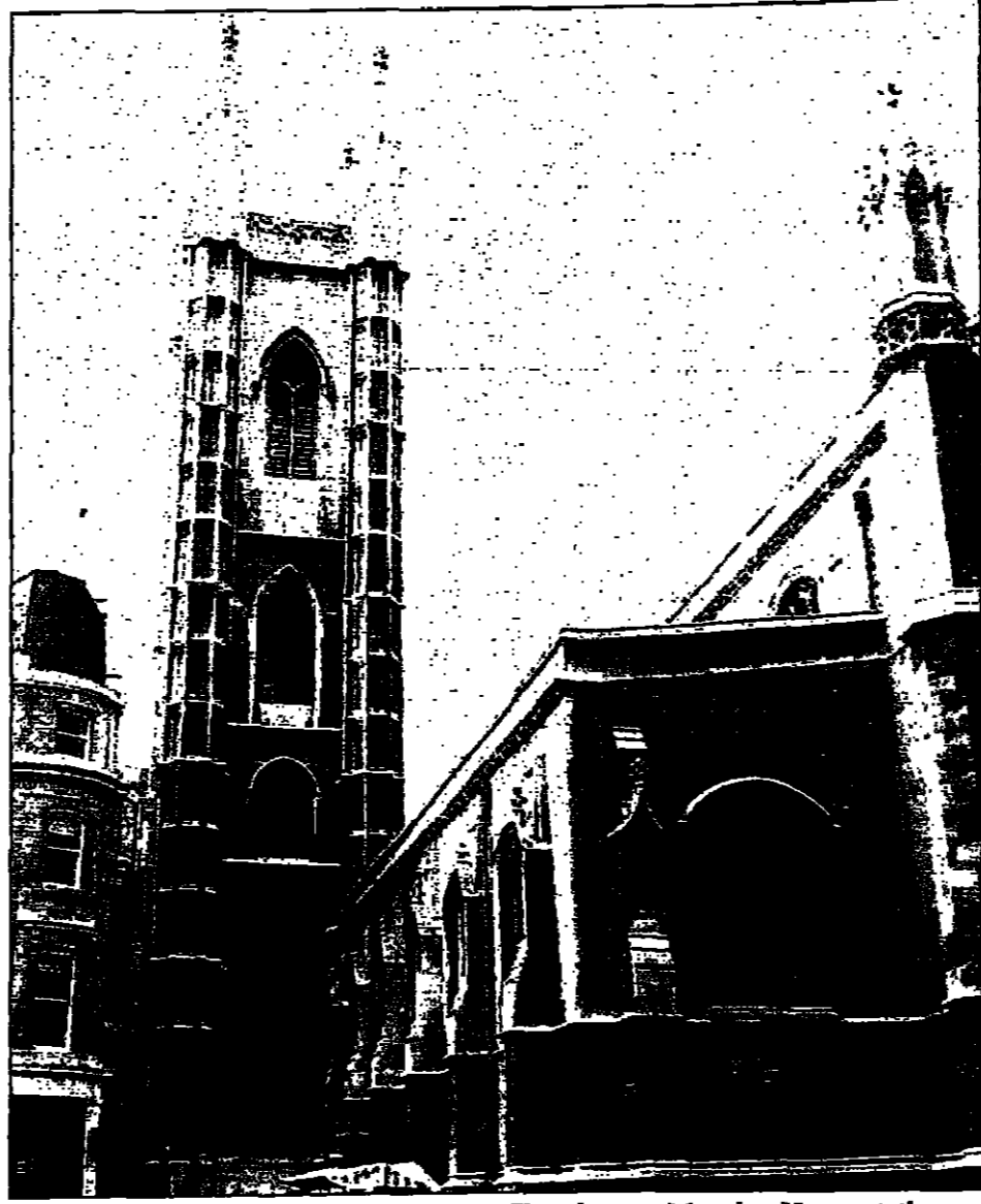
The walks start at St Mary Aldermary Church, near Mansion House station
